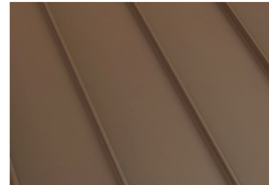
Copper standing seam roofing
