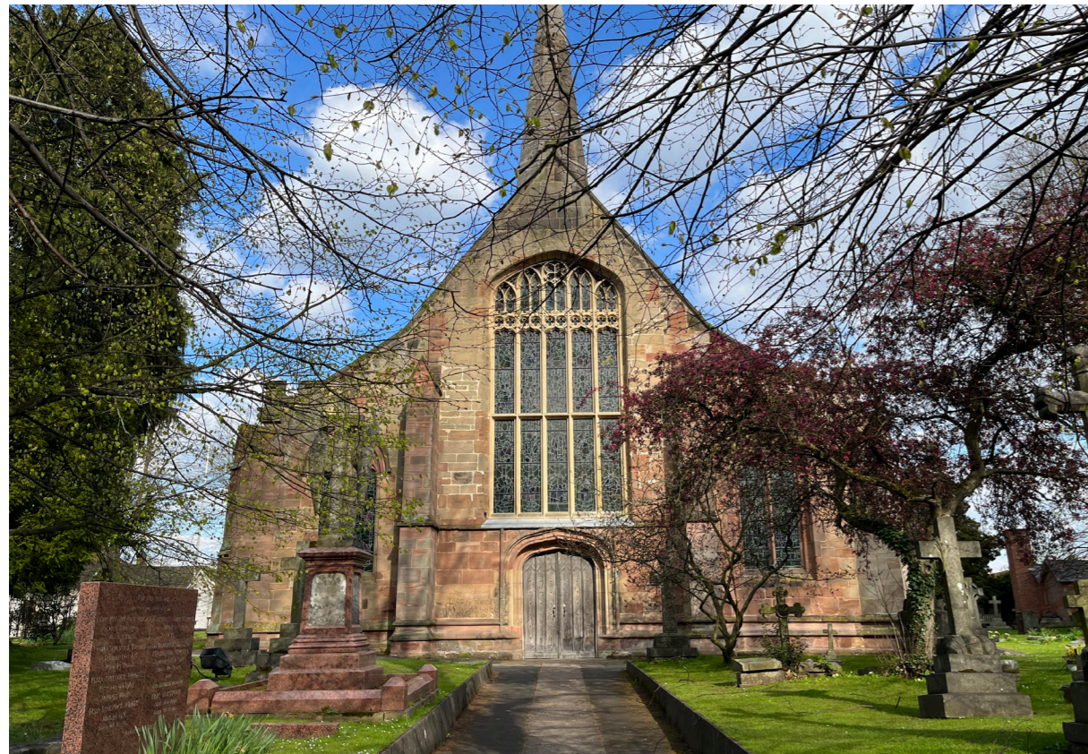
West entrance as existing
