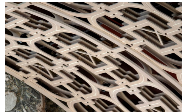
Perforated timber soffit
