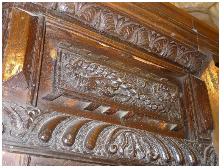
Figure 4. Detail of pulpit panel showing missing applied frieze pieces and woodworm damage.
