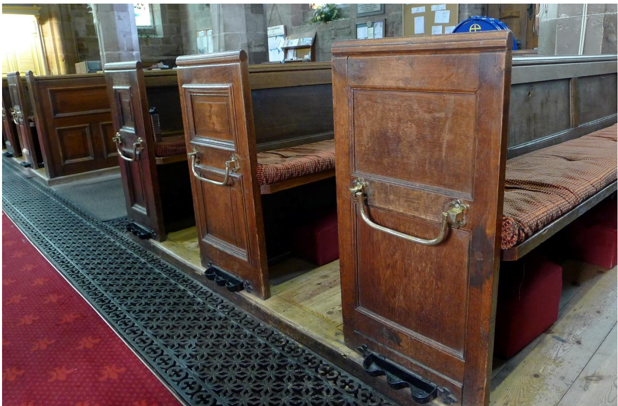
Figure 7. Bench-ends on the north side of the central aisle showing stained dowels.
