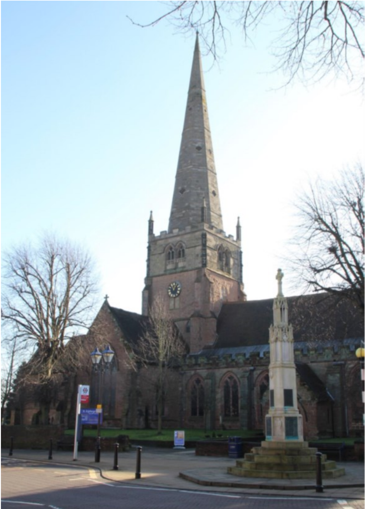
Exterior view of the church, showing the spire, north elevation and transept and war memorial.
