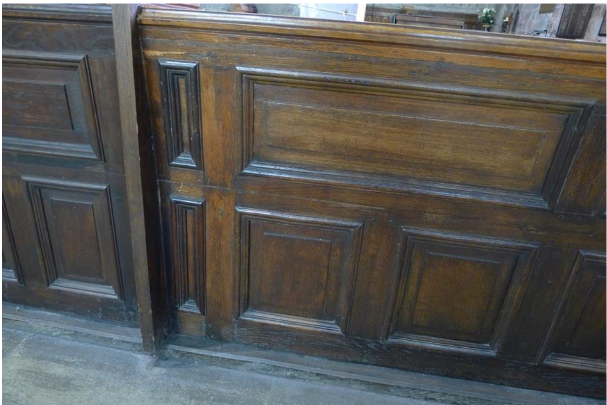
Figure 13. Rear of pews row showing re-working of older panelling to fit.
