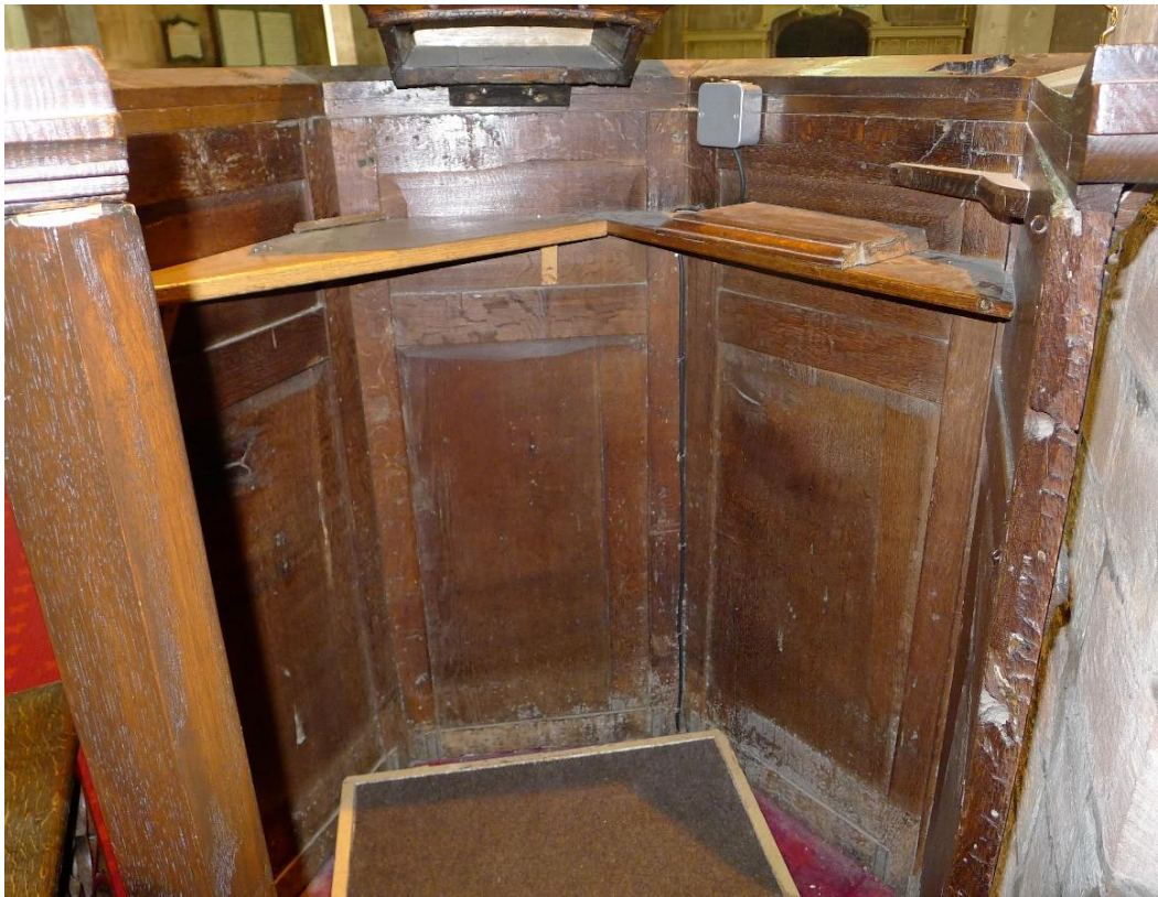
Figure 5. Interior of pulpit showing rear of panels, added top moulding, shelves and bible-rest.
