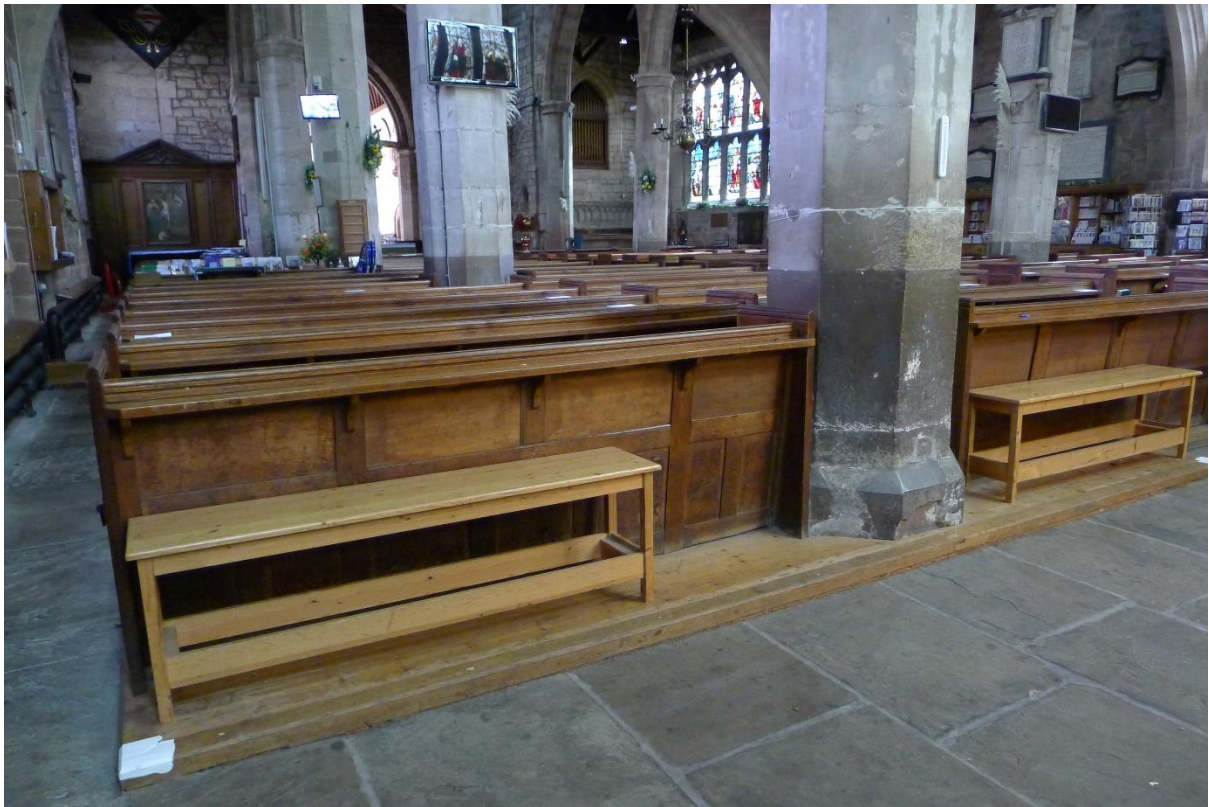
Figure 9. Pews in north aisle viewed from the rear of the nave.
