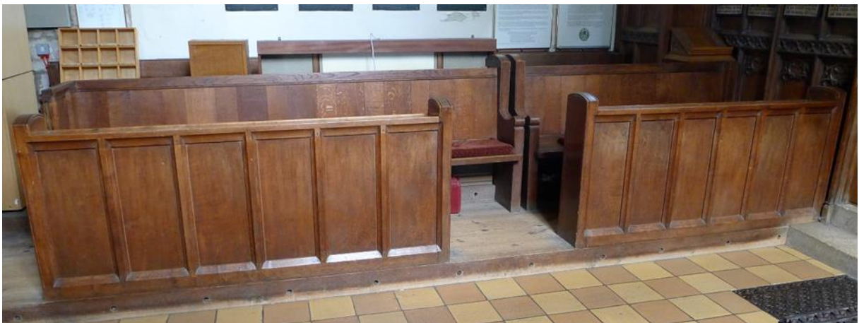
Figure 14. Chapel pews from the front showing mitred panels.
