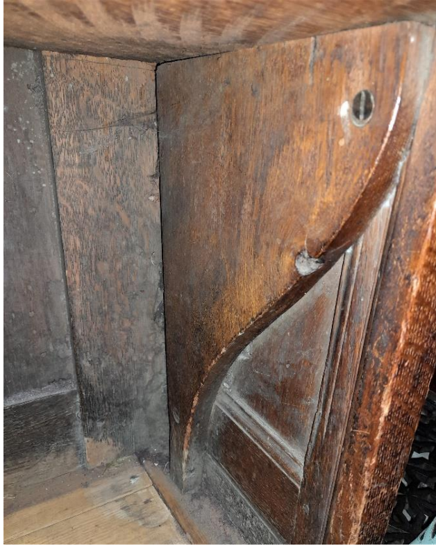
Figure 15. Additional support bracket beneath seat concealing panelled bench-end.
